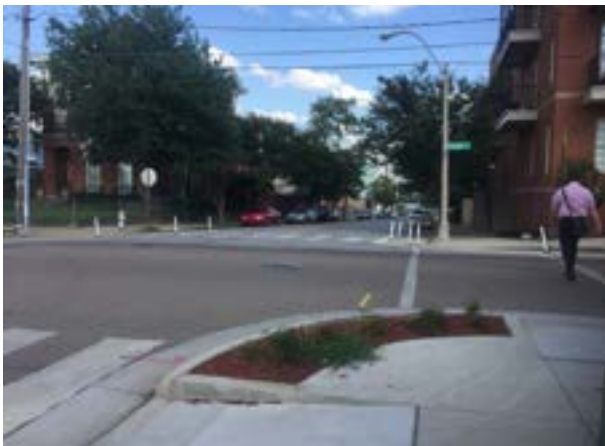
Tightened curb radius at pedestrian crossing
