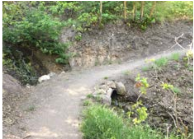
Small culvert at trail crossing
