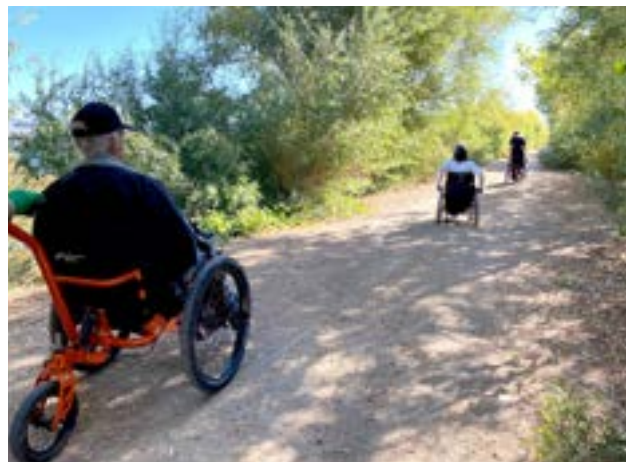
Crushed stone multi-use trails are flat, compacted, and accessible by a wide range of users (Trail Access Project).
