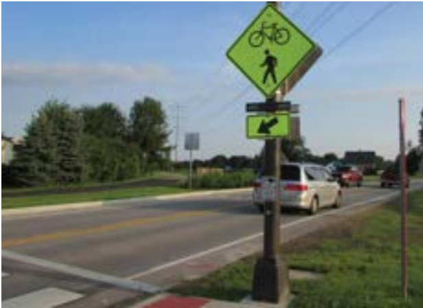
Flashing beacon with push button
