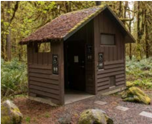
Backcountry Restroom - Vault toilet with structure (NPS)
