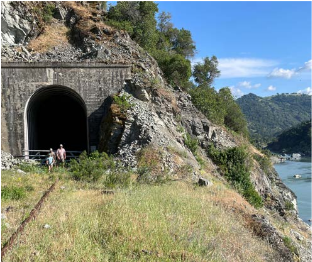
An existing tunnel along the Eel River Canyon.
