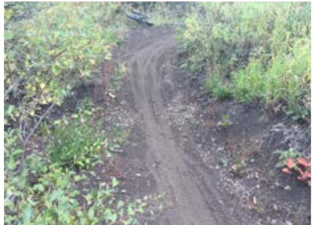
Dirt Crossings - drainage sheet flows across trail
