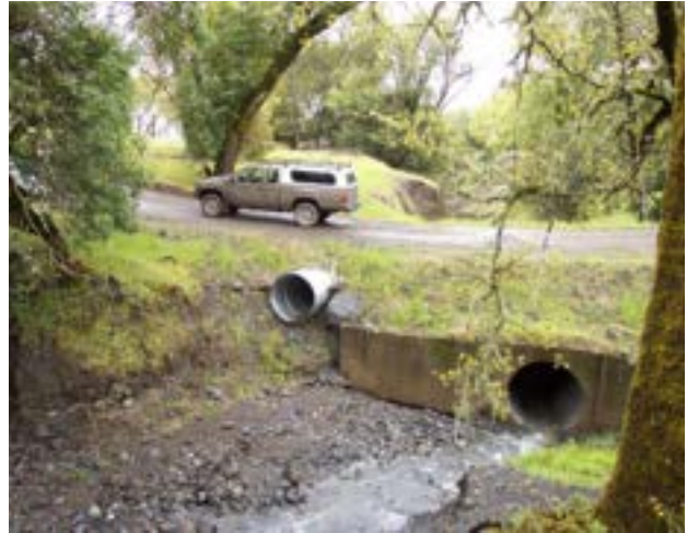
Emergency overflow culvert next to primary culvert
