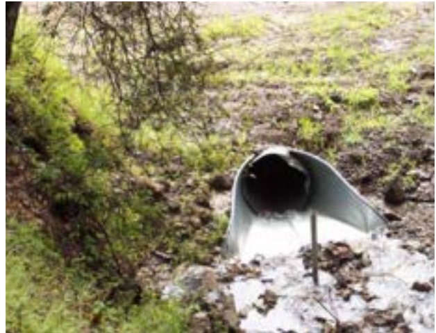
Flared culvert inlet
