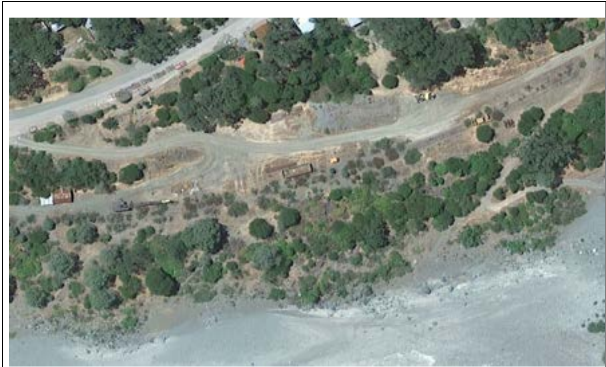
Photo 7 Image from Google Earth of the railroad debris and abandoned equipment located at the Dos Rios Road Site.
