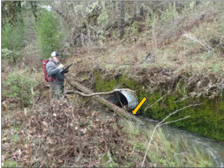
Photo 6. View of debris that blocked the stream crossing culvert inlet at MM 135.5 located on Walker Creek located on the Great Redwood Trail approximately 3.2 miles south of Willits, California. PWAs culvert sizing analysis determined that the culvert is not properly sized to convey the 100-year peak storm flow, including expected sediment and organic debris in transport. Arrow points to a log that floated into stream crossing and blocks culvert inlet.
