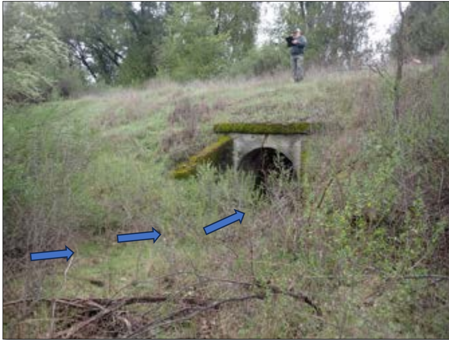
Photo 1. View of concrete culvert inlet at MM 108.5 a stream crossing culvert, on the Great Redwood Trail approximately 4.3 miles south of Ukiah, California. Arrows show flow direction. PWA estimated the 100-year peak storm flow rate at approximately 68 cubic feet per second (cfs) and determined that the existing culvert is properly sized to convey the 100-year peak stream flow including expected sediment and organic debris in transport.
