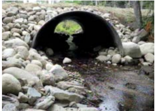
Arched Culvert with Stream Bottom
