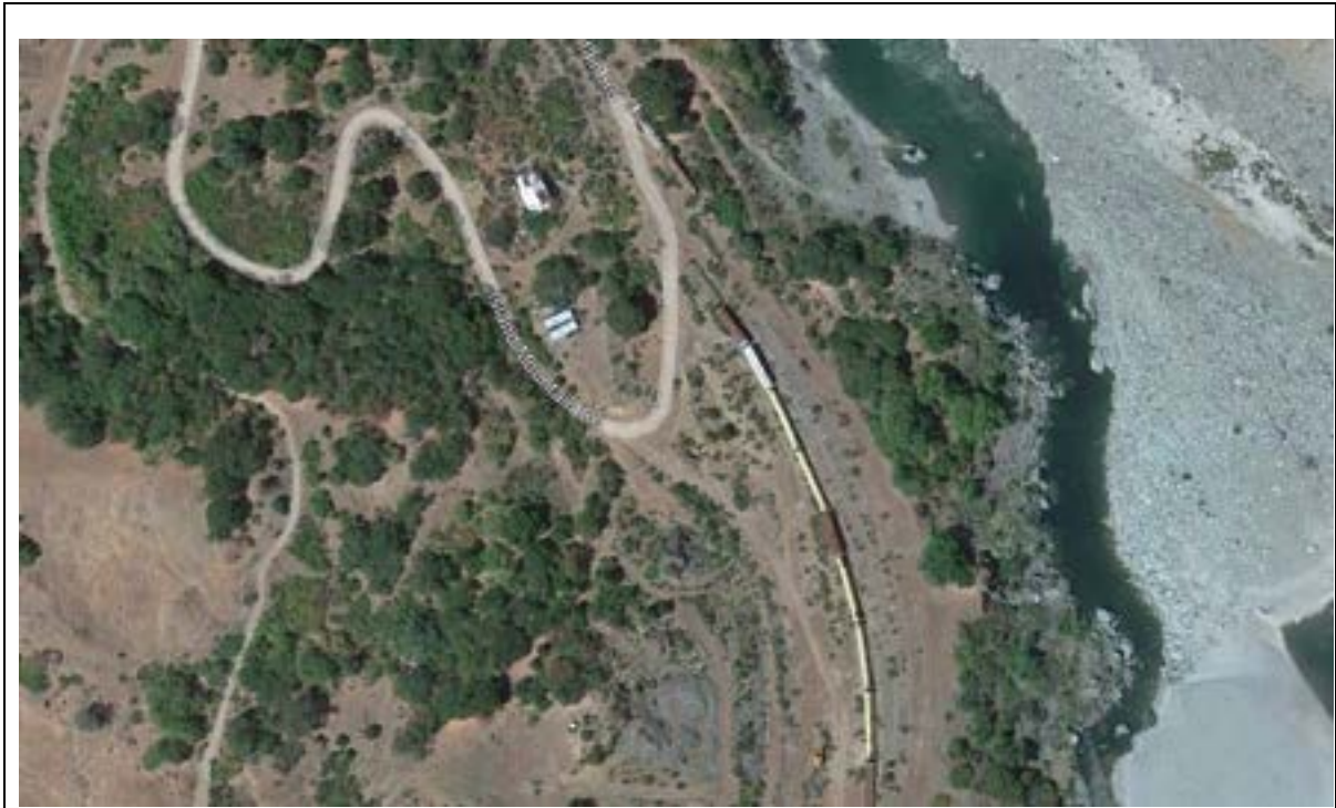
Photo 5 Image from Google Earth of the railroad debris and railcars located at the Island Mountain site.
