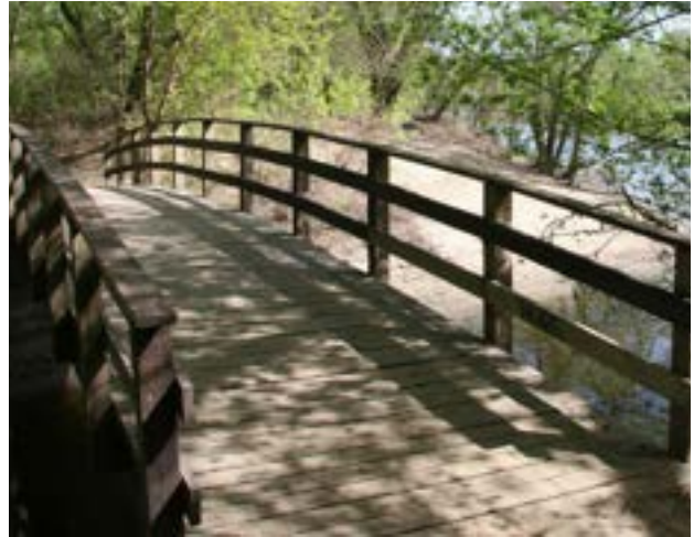
Bridge over Creek
