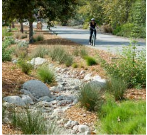
Bio-swale along a trail
