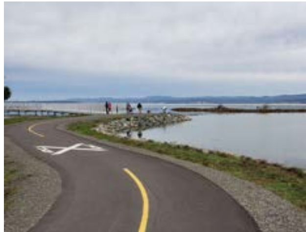
Paved multi-use trail (Existing in Eureka)
