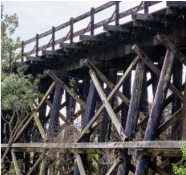
Existing trestle in Loleta
