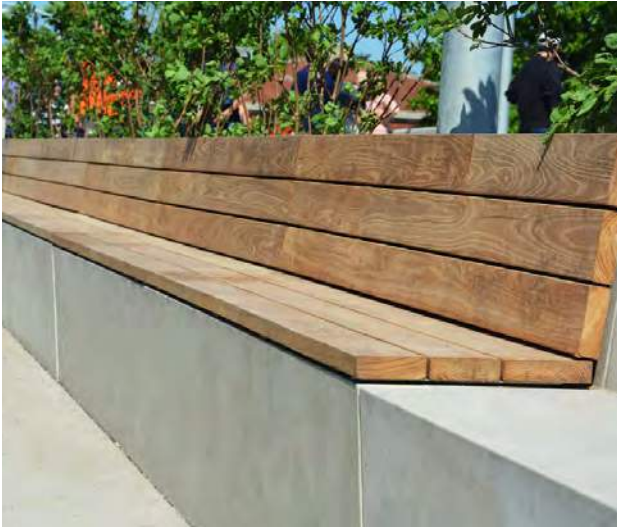
Seatwalls with wood toppers provide a durable and customizable option for community gateways and trailheads
