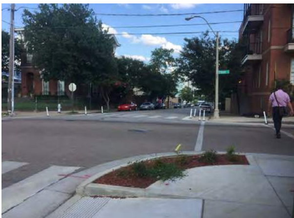
Tightened curb radius at pedestrian crossing
