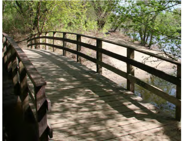
Bridge over Creek
