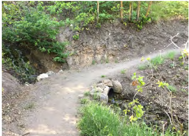
Small culvert at trail crossing
