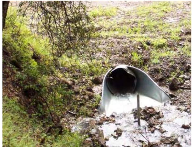
Flared culvert inlet
