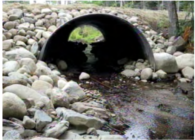
Arched Culvert with Stream Bottom
