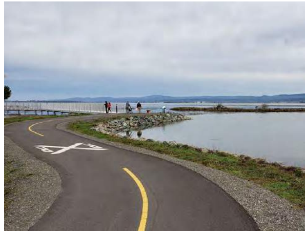
Paved multi-use trail (Existing in Eureka)
