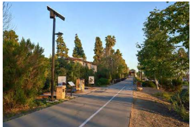
Solar lighting along a trail
