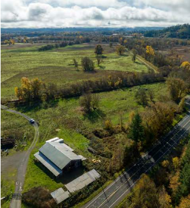
Overgrown GRT corridor in background, north of Willits
