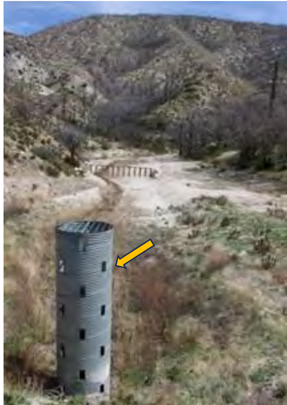
Photo 5. View of a vertical riser on a culvert inlet, usually of the same diameter as the culvert, and often slotted to allow water to flow into the culvert as streamflow rises around the outside. Drop inlets are often used on stream or ditch relief culverts where sediment or debris would otherwise threaten to plug a traditional horizontal inlet (Weaver et al., 2015).
