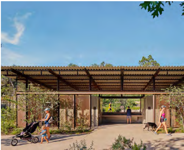
Developed Area Restroom - Flush toilets with integrated shade structure
