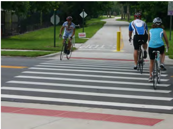
Tactile warning strips at curb ramp
