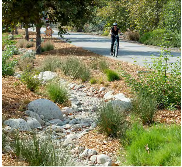
Bio-swale along a trail
