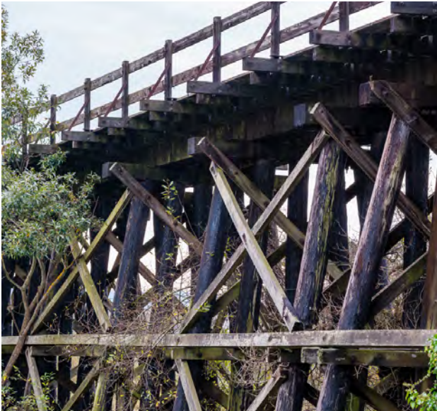
Existing trestle in Loleta
