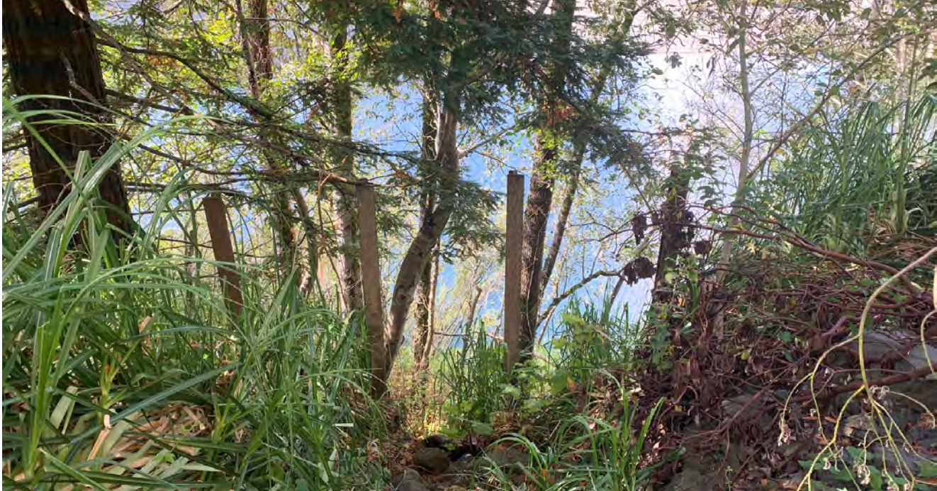
Washout of corridor with suspended track
