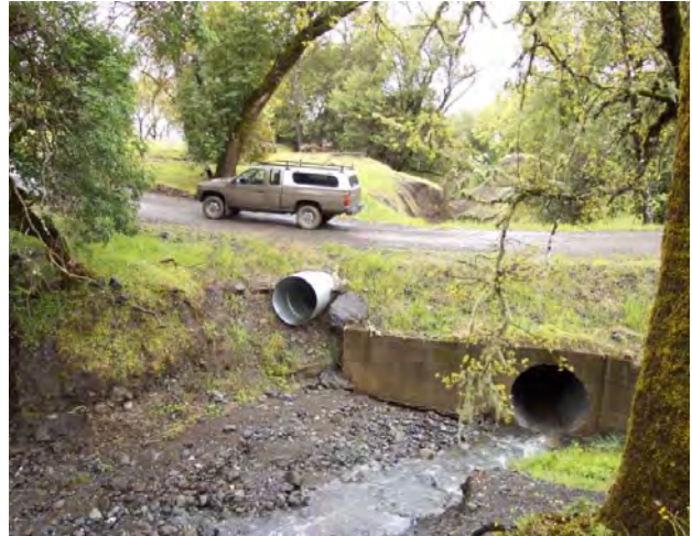
Emergency overflow culvert next to primary culvert
