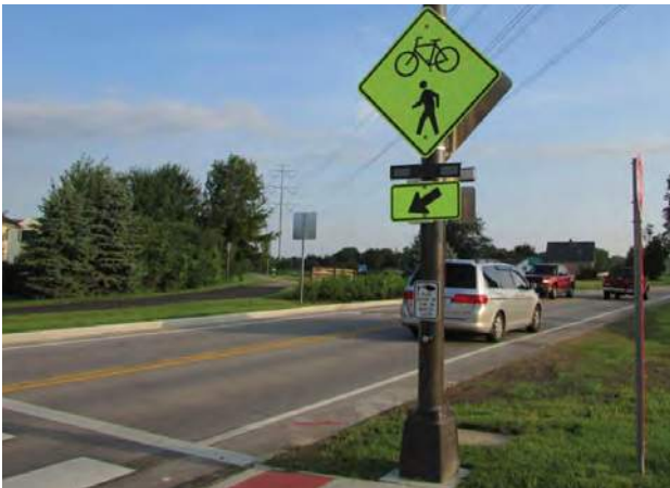
Flashing beacon with push button
