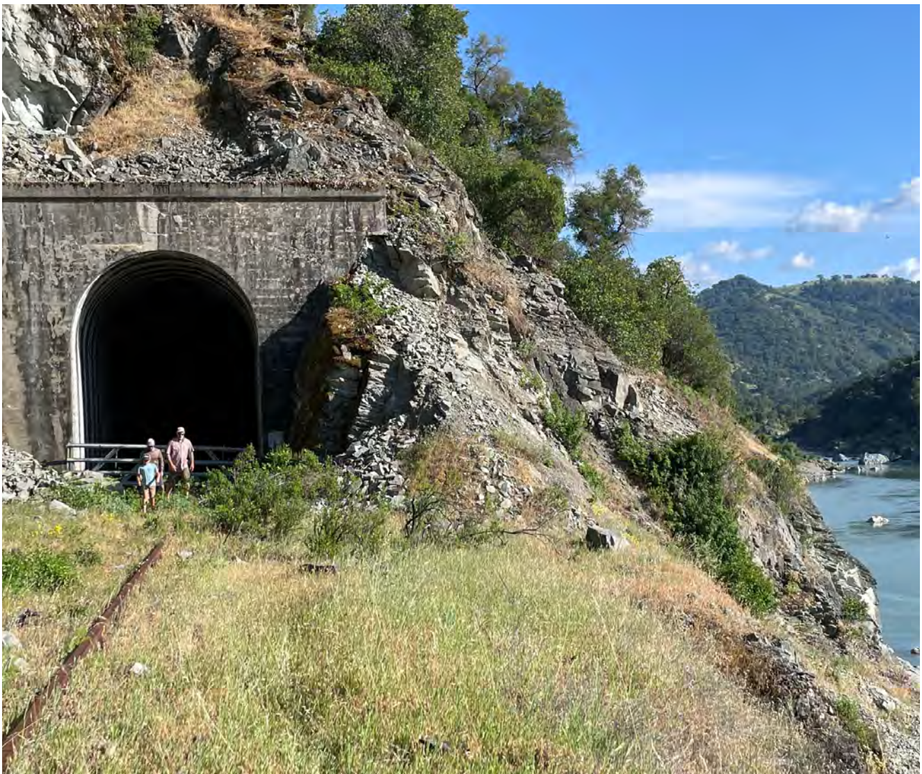
An existing tunnel along the Eel River Canyon.
