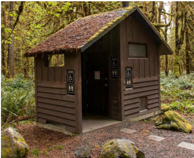
Backcountry Restroom - Vault toilet with structure (NPS)
