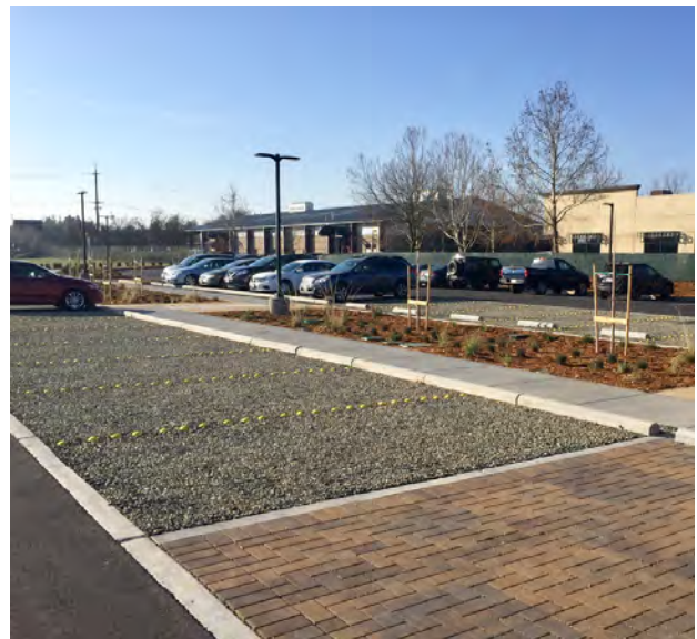
Pervious materials including pavers and pervious asphalt may be used for parking lots and driveways at trailheads
