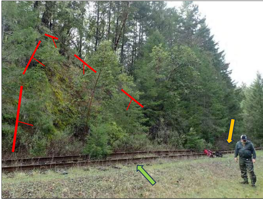
Photo 4. View of cutbank landslide (basic shape of main scarp is outlined in red) that plugged DRC (yellow arrow) and buckled tracks (green arrow) at MM 132.5 on the Great Redwood Trail. The cutbank landslide appears to have failed approximately 20 years ago based on the age of Douglas fir trees on the landslide deposit, which are 15 to 20 years old (basic shape of main scarp is outlined in red). The majority of the landslide is inactive, although a small rock fall occurred near the top in the recent past. The railroad tracks and wooden ties are slightly buckled and a little twisted.
